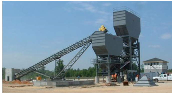
The new Wilson's Mills concrete plant
