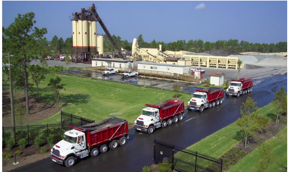
The new asphalt plant, which went online in March, is already bringing in big new jobs.
